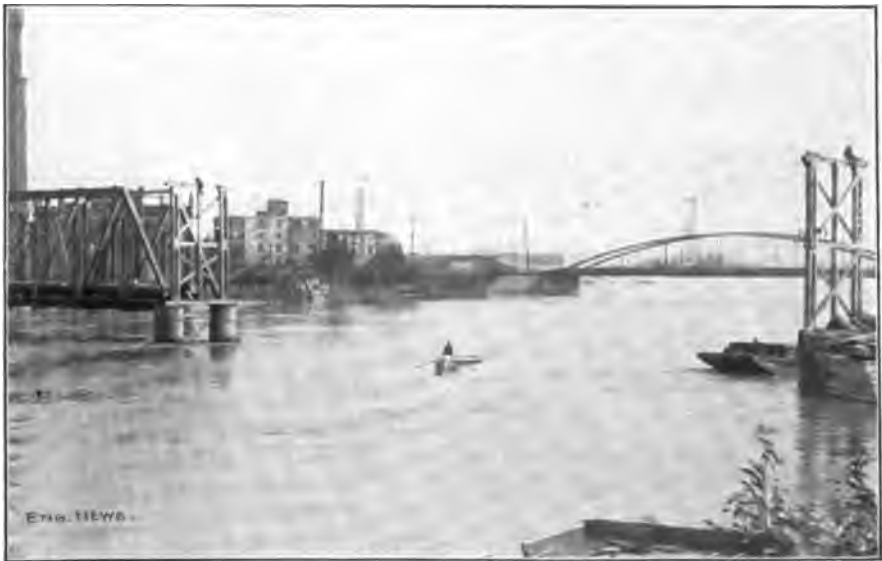
FIG. 3. VIEW SHOWING TIMBER BENTS ERECTED FOR FLOW-LINE SUSPENSION SPAN. (SPAN OF JAMES ST. BRIDGE IN THE BACKGROUND.)
